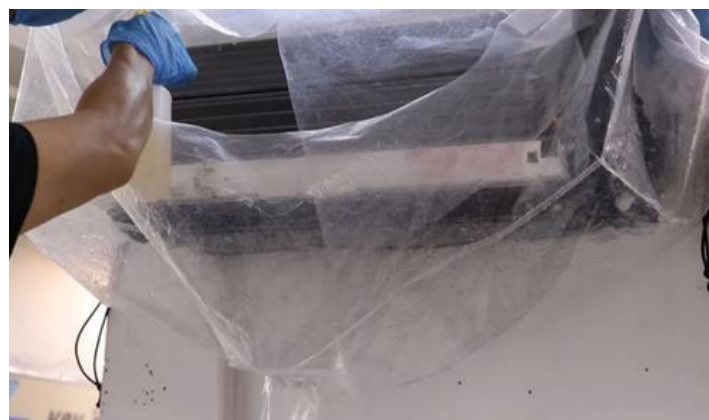
4. 安裝冷氣機污水收集袋以及噴上澳洲環保清潔劑 Multi-Enzyme HVAC Coil Cleaner
